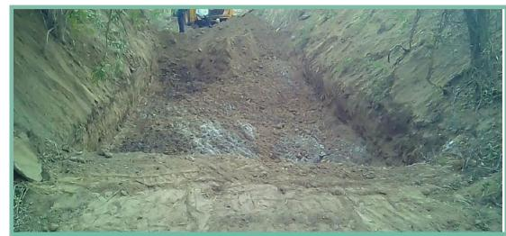
De-silting of a check dam at Chikla village of Dongri cluster. 1665 cubic meters of silt was removed.
