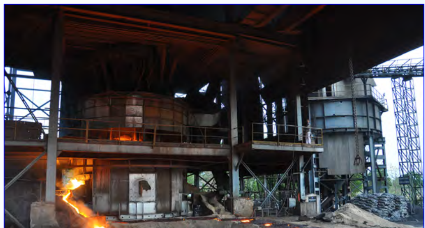
Tapping of molten metal at Ferro Manganese Plant at Balaghat
