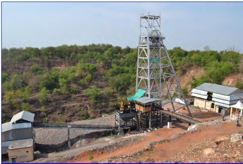
Vertical shaft at Gumgaon Mine
